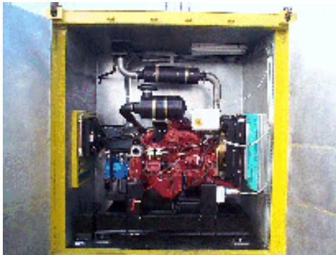
Acoustic Power House
