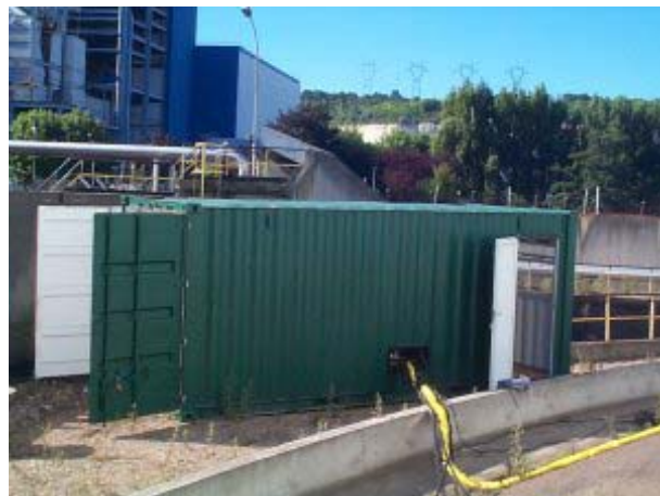
Container with power pack and control room
