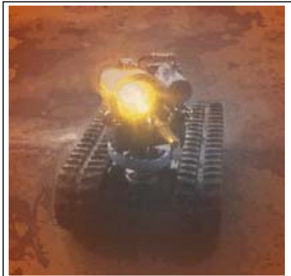
ROVERjet INSIDE CLEANED TANK
